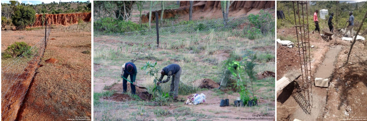
Learning skills and gaining experience - restoring eroded land, planting trees, putting in foundations
