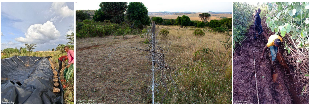
Building a dam, regeneration of savanna grassland and laying water pipes.
